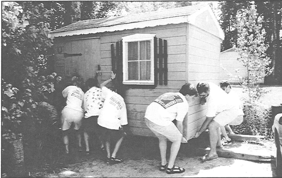
The new Youth Sailing storage building is moved into place at the WYC Yard
